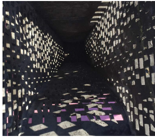
Building three hollow columns from above
