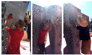
Building last lightweight column with only 2 people
