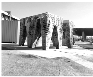
One more column left to install.
